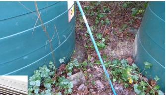
Product (kerosene) was visible in high concentration around the base of both tanks, in pooled ground water.
