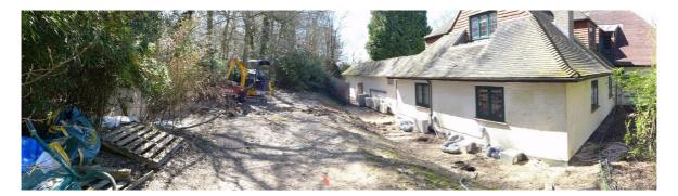
Excavations were to a depth of 1-1.5m and removed approximately 70tonnes of soil during the full excavation phase of this claim.
