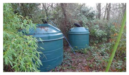
Originally a 2,500 litre tank was present (the right hand tank) and following the construction of the swimming pool and the oil being used too quickly a second 5,000 litre tank was installed.
