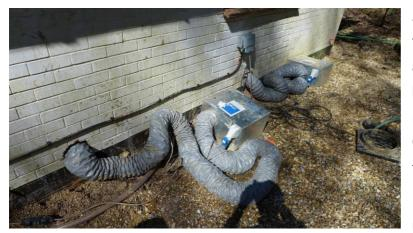
A vapour extraction kit was installed in the main dwelling, in order to promote air-exchange to reduce the odour that kerosene gives off; the odour is referred to as Volatile Organic Compound (VOC) and is measured in this unit of reference.
