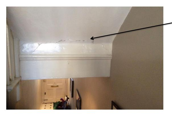
Cracks under the stairs near Party Wall
